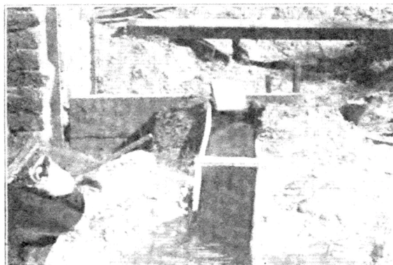
Fig. 32. Discharge of about 450 gallons per minute through a six-inch pipe from pump of J. Stoney Porcher, El Paso, Texas.
